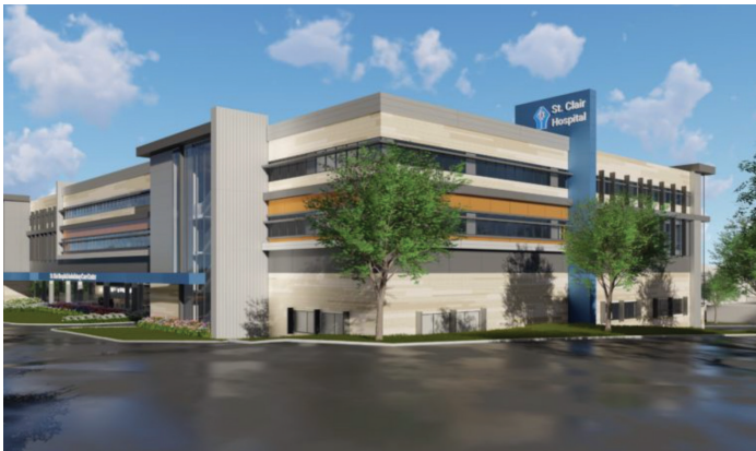
Architectural CMU dresses up the 280,000-square-foot Dunlap Family Outpatient Center, which opened in the spring of 2021.
